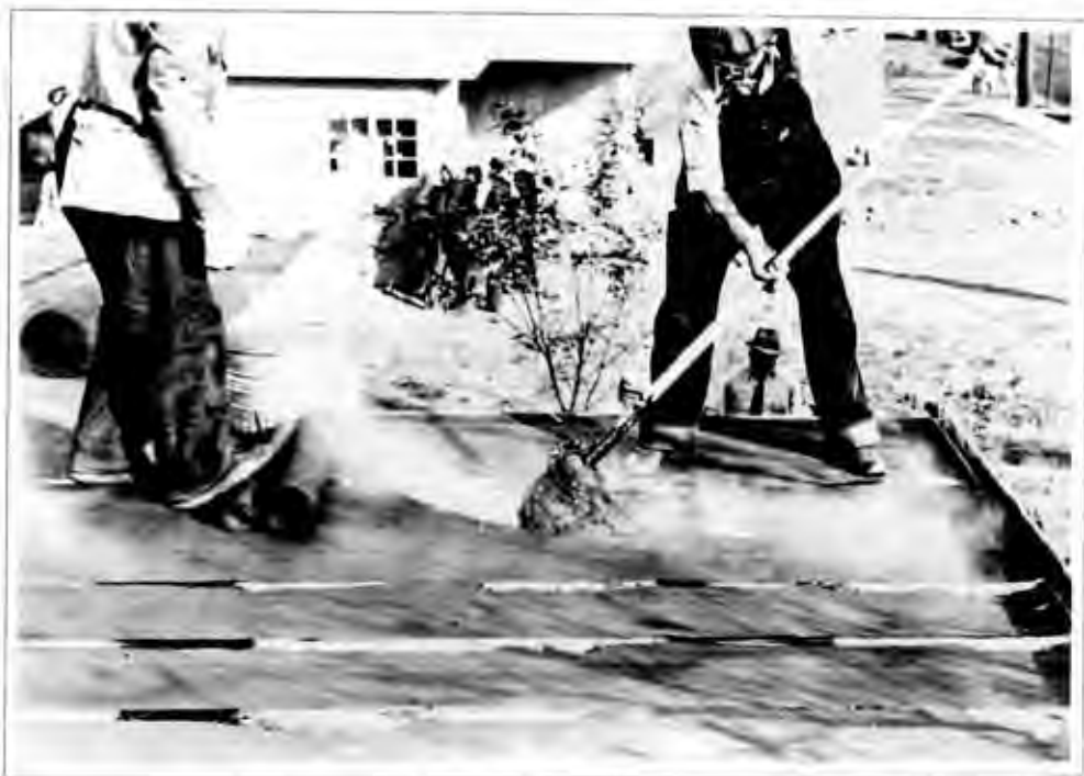
The roof is dead level. A four-ply pitch and gravel, seventeen-year specification roofing is applied. In calculating rents, this roof is written off on a ten-year basis.
