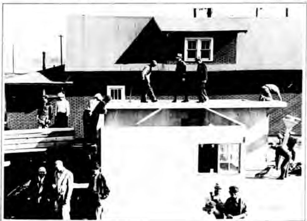
These are finished panels sufficient to make up the walls for four complete houses. Below is a house under construction with all the wall panels in place, and the roof panels being set.
