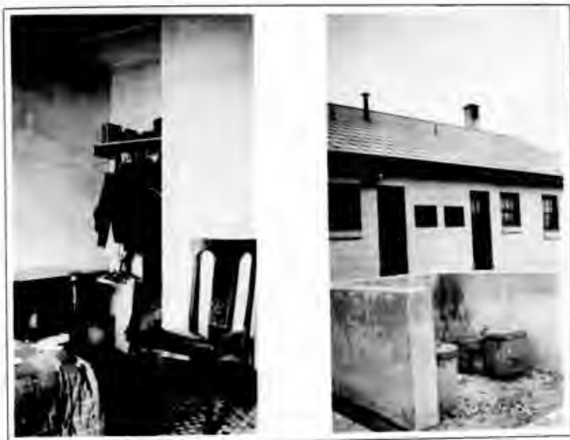
The left-hand photograph shows a typical recessed open closet. Note the rod provided for a curtain. The right-hand photograph shows the concrete waste receptacles. The two doors in the house are to utility rooms provided for each dwelling unit. They contain a coal bin, hot water heater, and the bathroom plumbing pipes.
