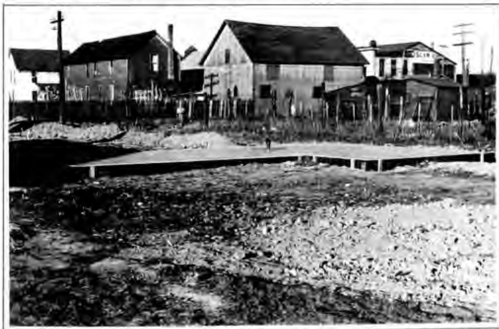
The floor is formed by a concrete mat reinforced with wire mesh and laid over gravel. With this construction, the floor assumes equable earth temperature and is warmer in winter and cooler in summer than if it were ventilated. The tenants, when questioned, said that the floor was not too cold in winter weather.
