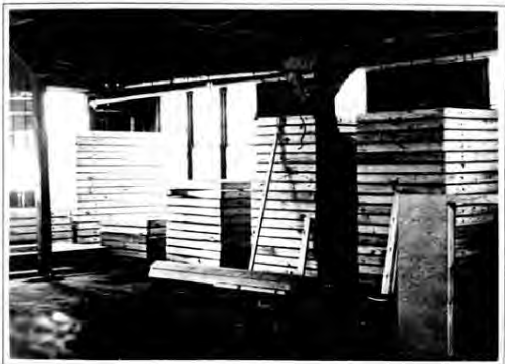
These are finished panels sufficient to make up the walls for four complete houses. Below is a house under construction with all the wall panels in place, and the roof panels being set.
