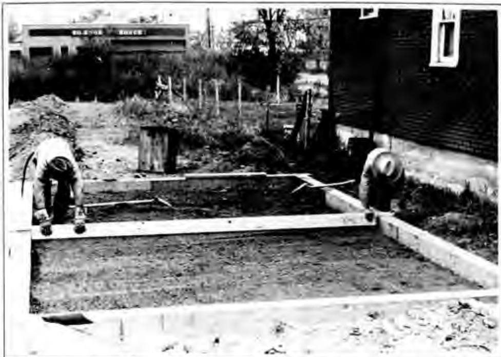
The floor is formed by a concrete mat reinforced with wire mesh and laid over gravel. With this construction, the floor assumes equable earth temperature and is warmer in winter and cooler in summer than if it were ventilated. The tenants, when questioned, said that the floor was not too cold in winter weather.
