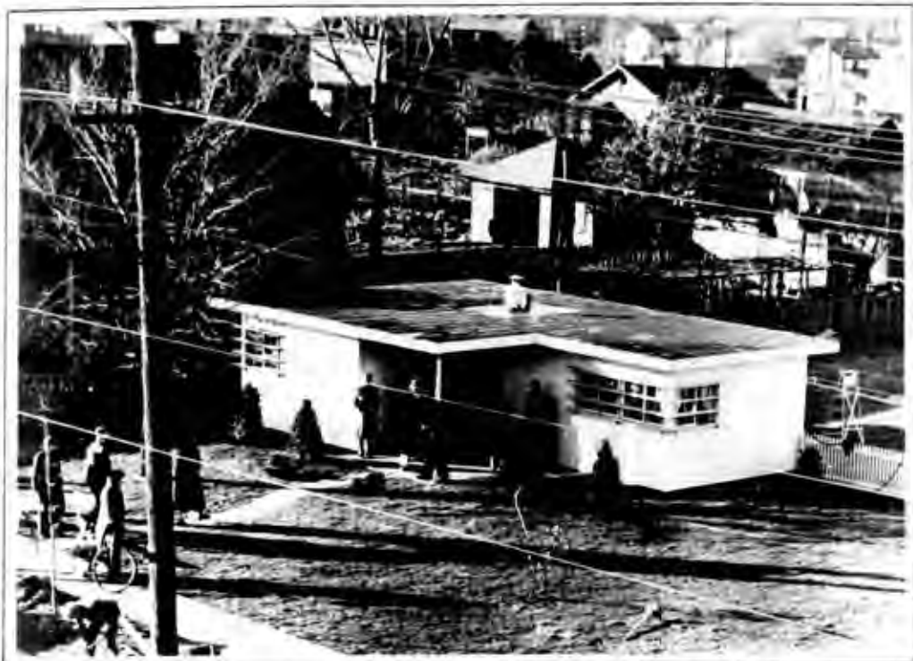
A typical Fort Wayne House. The shell of the house can be erected in two hours. It can be dismantled and moved to another site. The interior arrangements are shown in the plan and the model below. It will be noted that there is a large living room with one end equipped with kitchen equipment and heating stove. The two bedrooms are small, and are provided with open-front closets which may be entirely closed with curtains.
